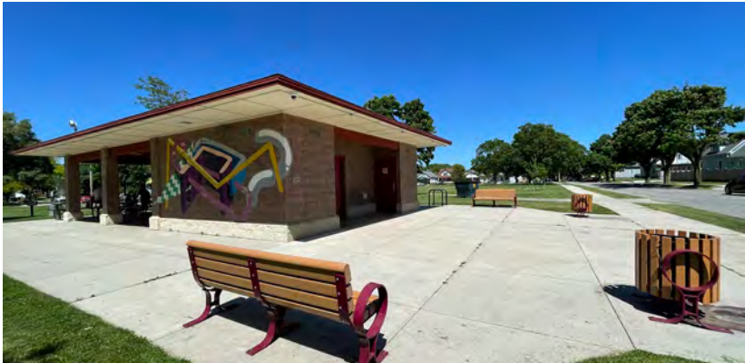
▲ End Park facility with benches.
