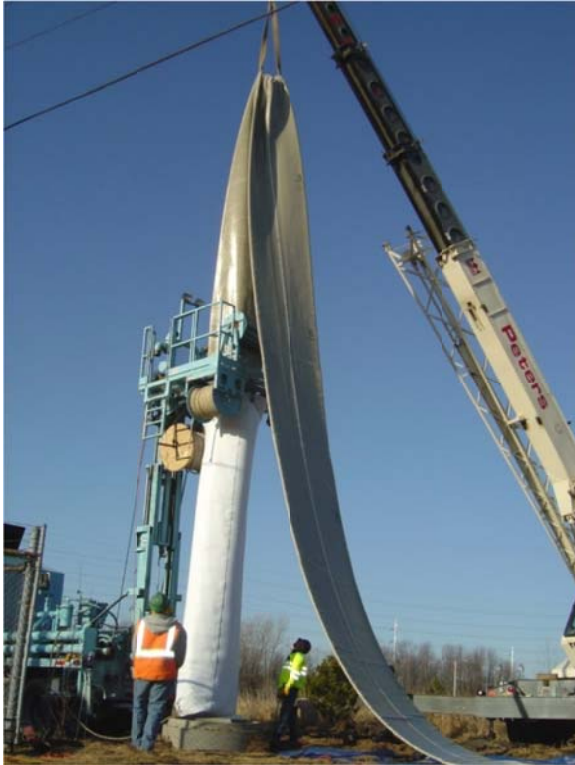
Liner Being Inserted Into Sewer Pipe
