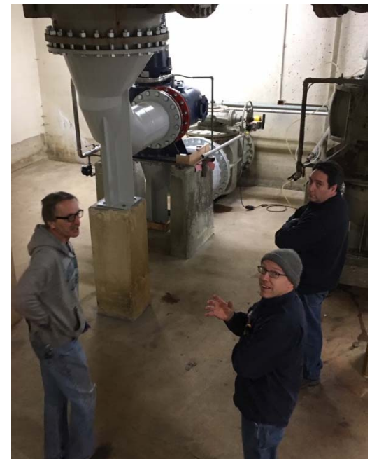
Installation of new Raw Influent Pump
