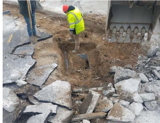
Storm Drain (Catch Basin) Installation
