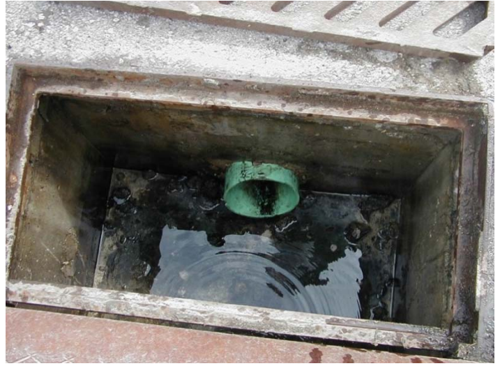
Catch Basin Cleaning, Before (Left) and After (Right)
