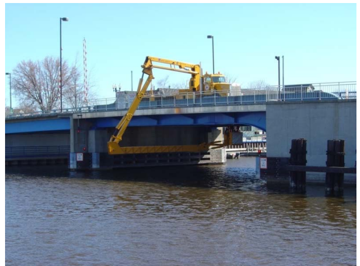
8 th Street Bridge being inspected
