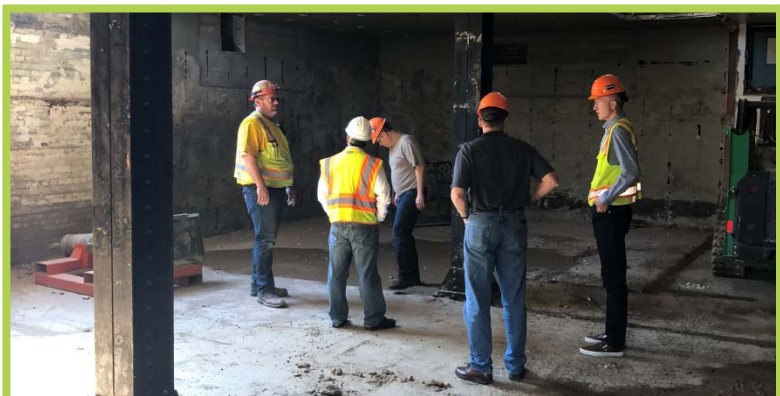
Basement Renovation in Progress at City Hall
