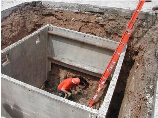
Preparing to Install a new Sanitary Manhole
