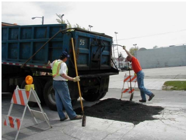
Street Excavation Patch
