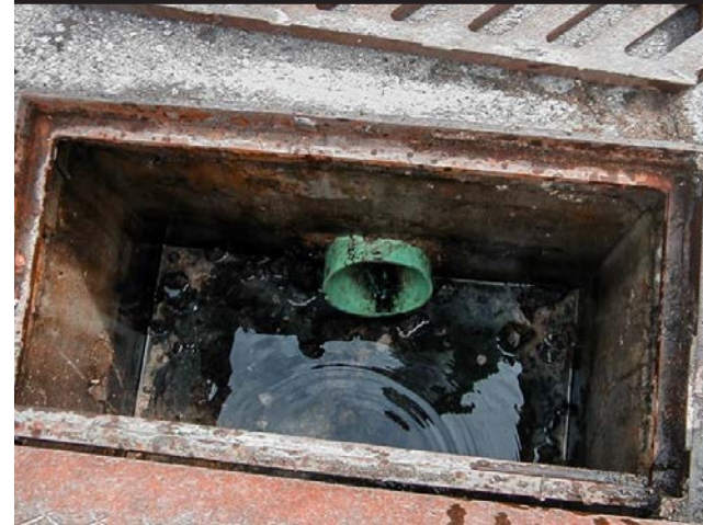
Catch Basin before and after cleaning
