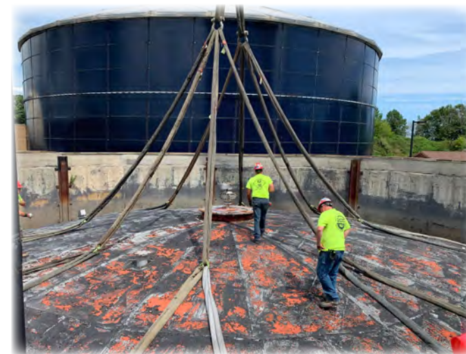
Cover on Digester #6 being rigged for lifting
