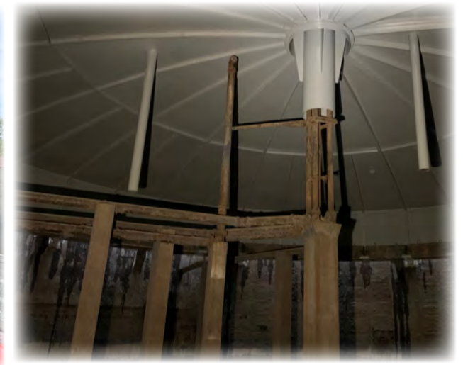
Cover on Digester #6 installed on the digester
