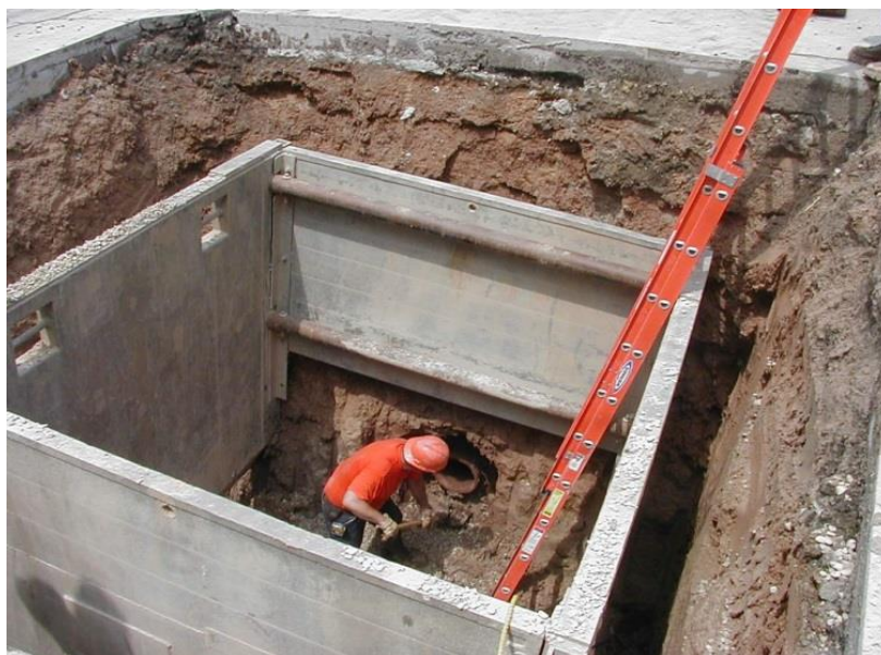
Preparing to install a new sanitary manhole
