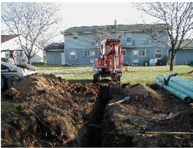
Mini-Storm Sewer Installation - Backyard
