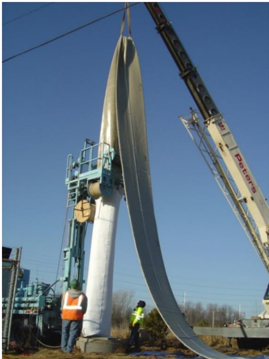
Liner Being Inserted Into Sewer Pipe
