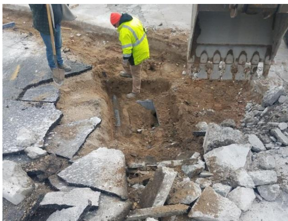
Storm Drain (Catch Basin) Installation
