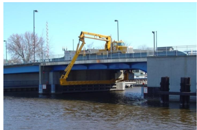
8th Street Bridge being inspected
