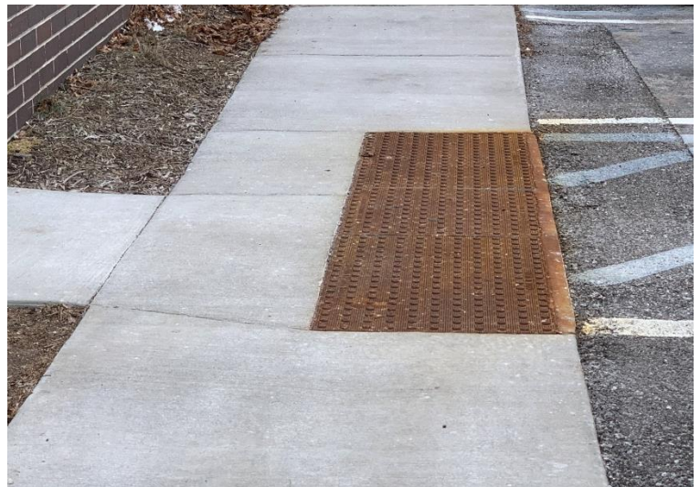
ADA Accessible Ramp outside of former Social Security Administration Building
