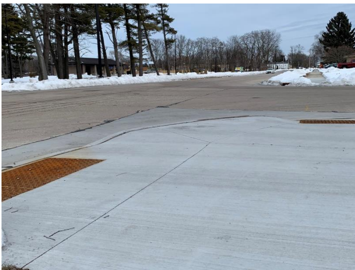
ADA Accessible Ramps near Shaw Family Playground
