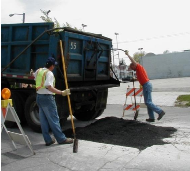
Street Excavation Patch
