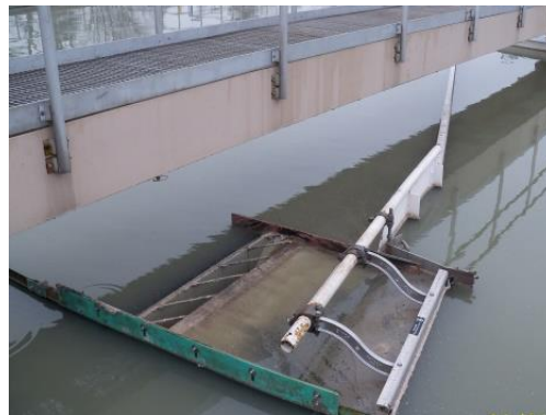
New Skimming Mechanism and Beach on Clarifier #2
