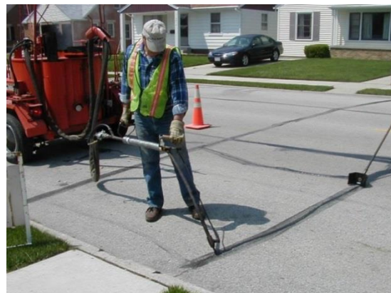
Crack Filling
