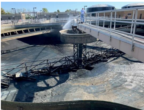
Operator Cleaning Clarifier #2
